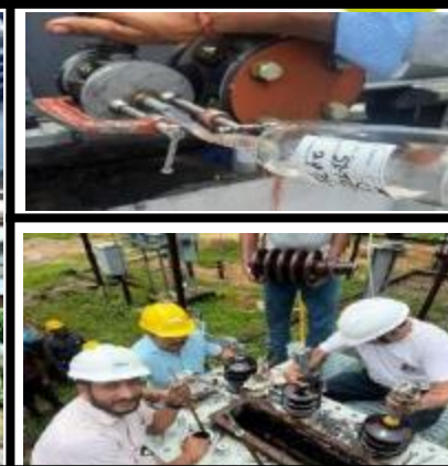
Inhouse DGA, Oil Filtration, PTR repairing Started
