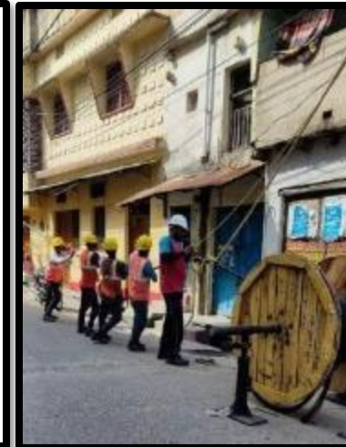
Bare conductor to AB cable replacement work
