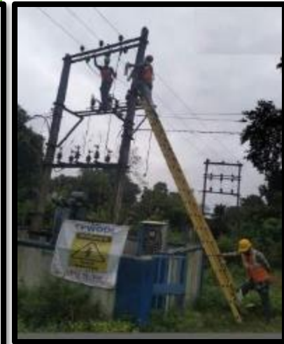
New AB switch installation work
