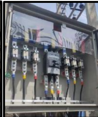
Feeder Pillar installation
