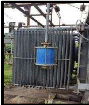
Project Neela: Ensuring Blue Silica gel in 100% PTR
