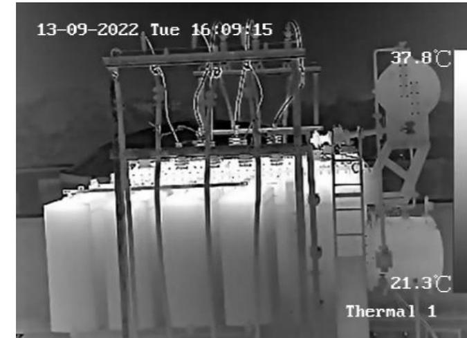
Real Time monitoring-Thermal View of EMC Park Substation Equipment
