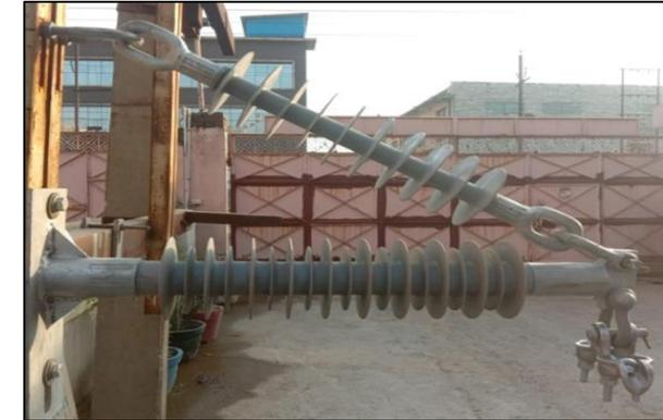
**Cross arm and insulator combined into one piece**
